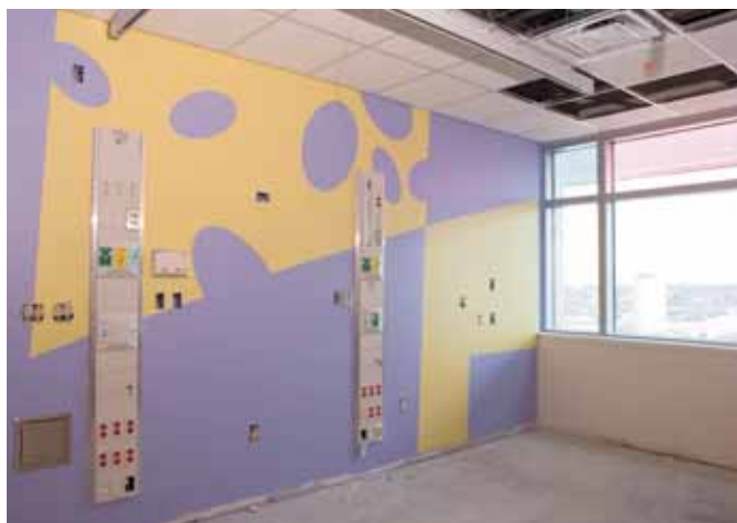
Children's Hospital room, under construction
