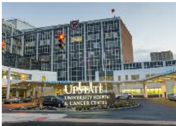
One of Upstate's most visible sustainability efforts includes the rainwater collection basin that was incorporated into the hospital traffic circle design. It will remove or divert more than 1 million gallons of rainwater from the city sewer system.
